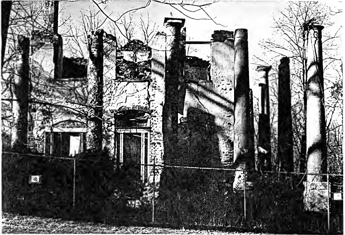
Figure 31: South elevation of Pawling/Wetherill House
